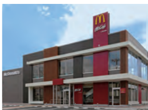
飲食店新築工事
